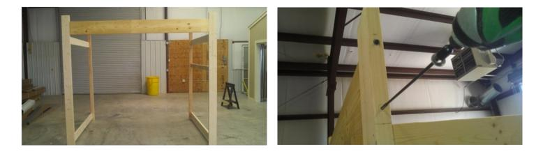
Fasten the front beam with 12" Deckmate lags
